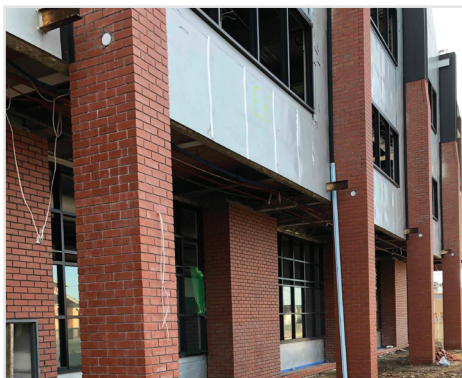
↑ External brick cladding advancing
