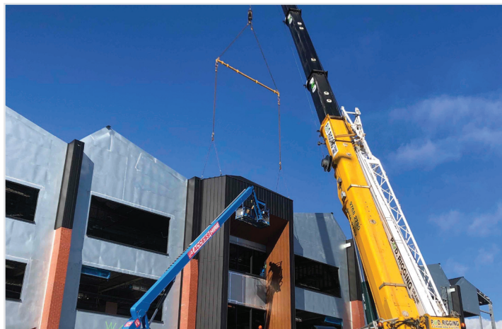
↑ One of the first modules installed onsite
