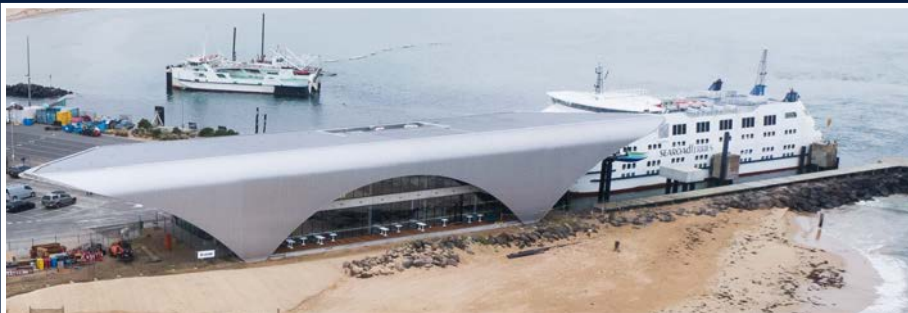
Redevelopment of Queenscliff Ferry Terminal
